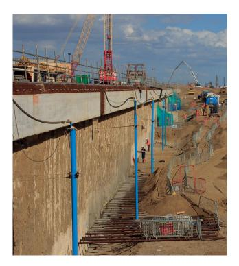
At the heart of each system an innovative electrical pump station is used to power and control multiple pumps from a central location. Control options include automatic mains failure (AMF) switchover to standby power, visual/audio/GSM text alarm systems, and a secure Cloud based data logger for monitoring groundwater flows, pressures and levels.
