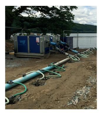
Pumping options include surface electric or diesel suction pumps and super-silenced models for residential areas.
